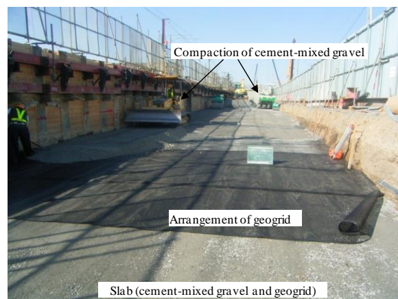
Figure 21. Application of cement-mixed gravelly soil slab to the construction of railway embankment on the soft ground
